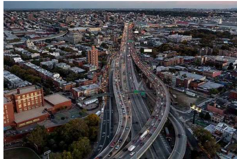
Figure 4: Brooklyn–Queens Expressway (USA)
