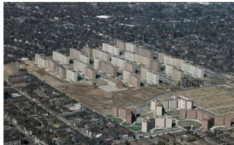
Figure 6: Pruitt–Igoe Housing, St. Louis
